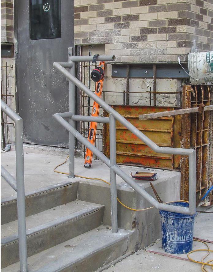
Concrete and Rebar Flood Walls
