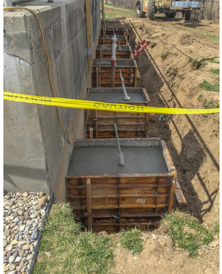
Helical Piles for strength against wave action
